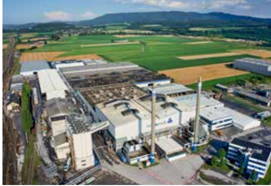
Pöchlarn Plant, Austria
